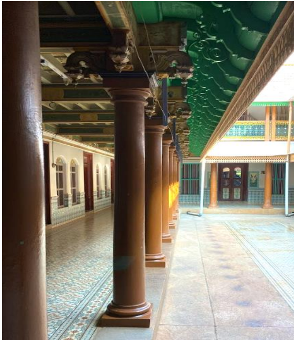
Fig 11: The overhanging eaves at Kanadukathan, Karaikudi, Tamil Nadu.
