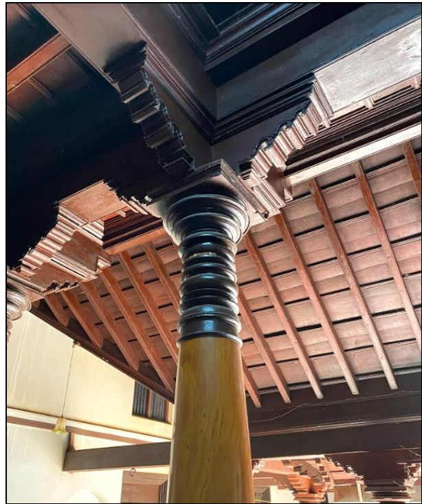
Fig 12: Detail of a pillar in CVCT House, Kanadukathan, Karaikudi, Tamil Nadu.
