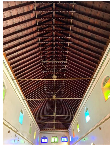
Fig 4: Burma teak wood ceiling in Athangudi palatial mansion, Athangudi, Karaikudi, Tamil Nadu
