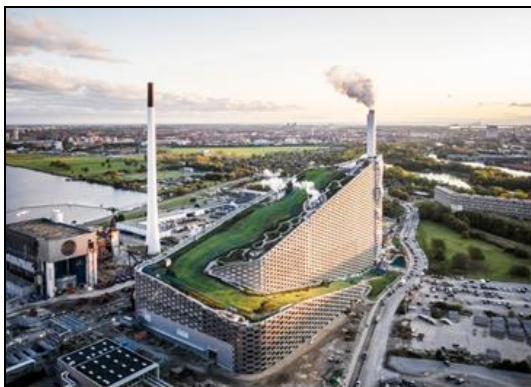
Fig 1: Aerial views of Copenhagen's CopenHill Waste-to-Energy Plant, showcasing its integration of urban utility and recreational spaces.
