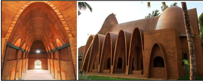
Fig 1: St. Gerge Orthodox Church, Chalakkudy, Kerala
